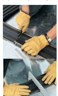
1. Always cut square ends before welding waterstops. Never weld to extruded ends.
