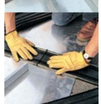
3. Quickly remove **Sireg Welding Blade** and gently press waterstops ends together until they bond (approximately 3 to 5 minutes or cool to touch). Cold water may be sprayed on waterstops to expedite the bond.
